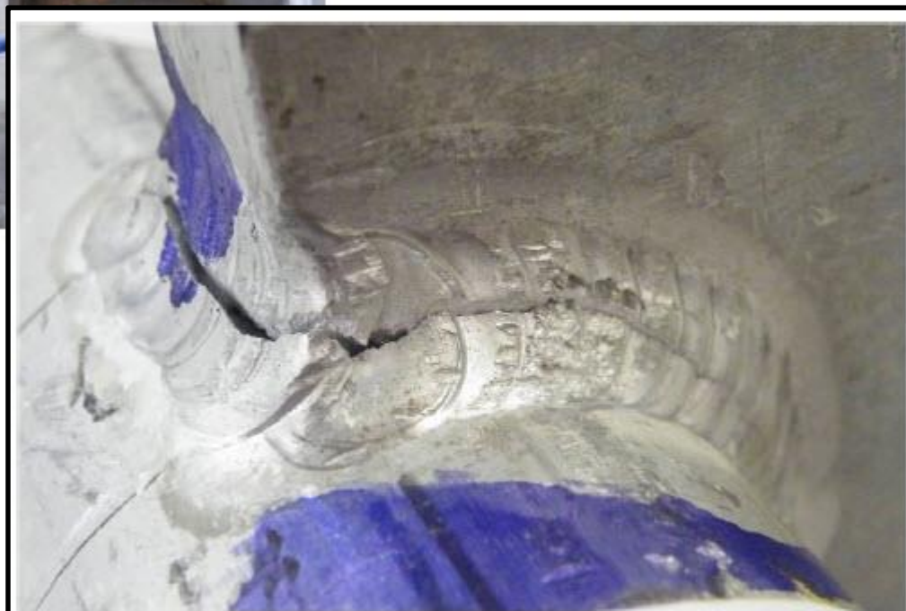
Fig. 8 Failure of fin plate F4 EAST
